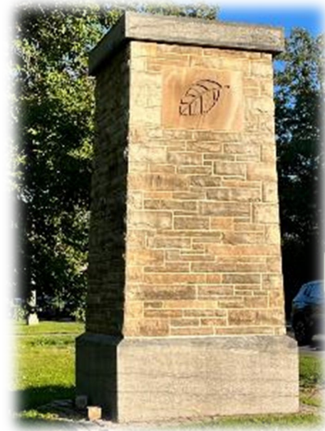
Figure 17: Repeating NCC stone cairns announcing Gateway to Island Park Drive entering IPD @ Ottawa River Parkway, and throughout Island Park Drive
