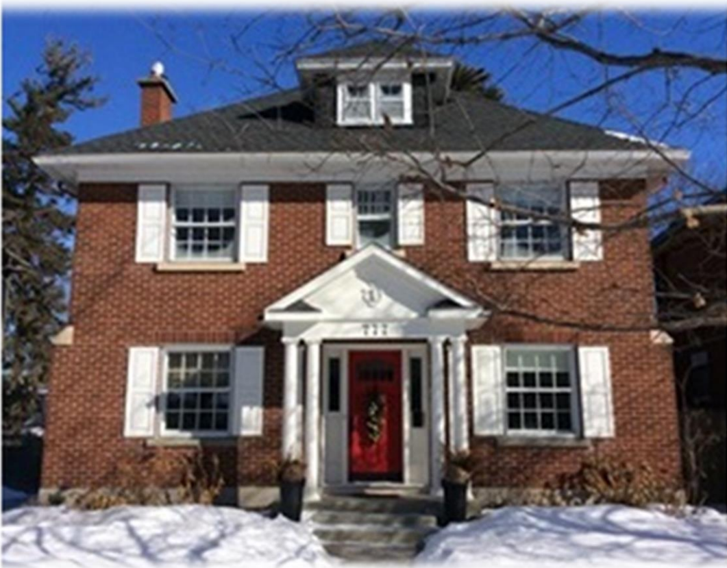
Georgian Revival 777 Island Park Drive – 1942
